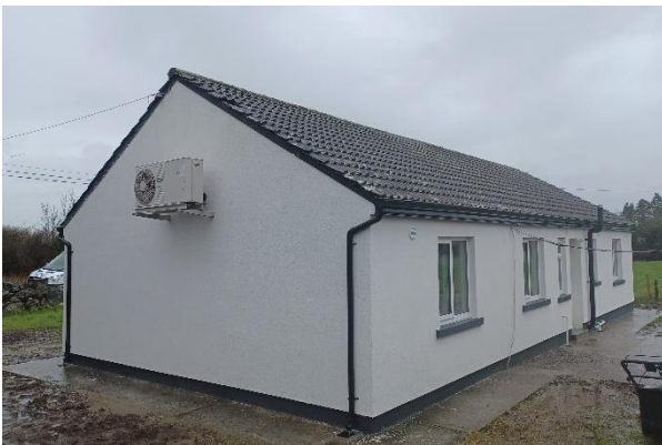
RURAL BUNGALOW SHOWING EXTERNAL INSULATION AND HEAT PUMP
