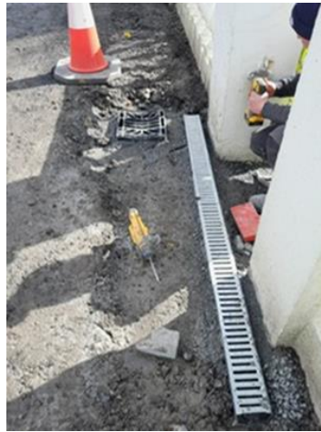
DRAINAGE WORKS AT KILCOOLEY ON THE N65 TO ALLEVIATE SURFACE WATER FLOODING
