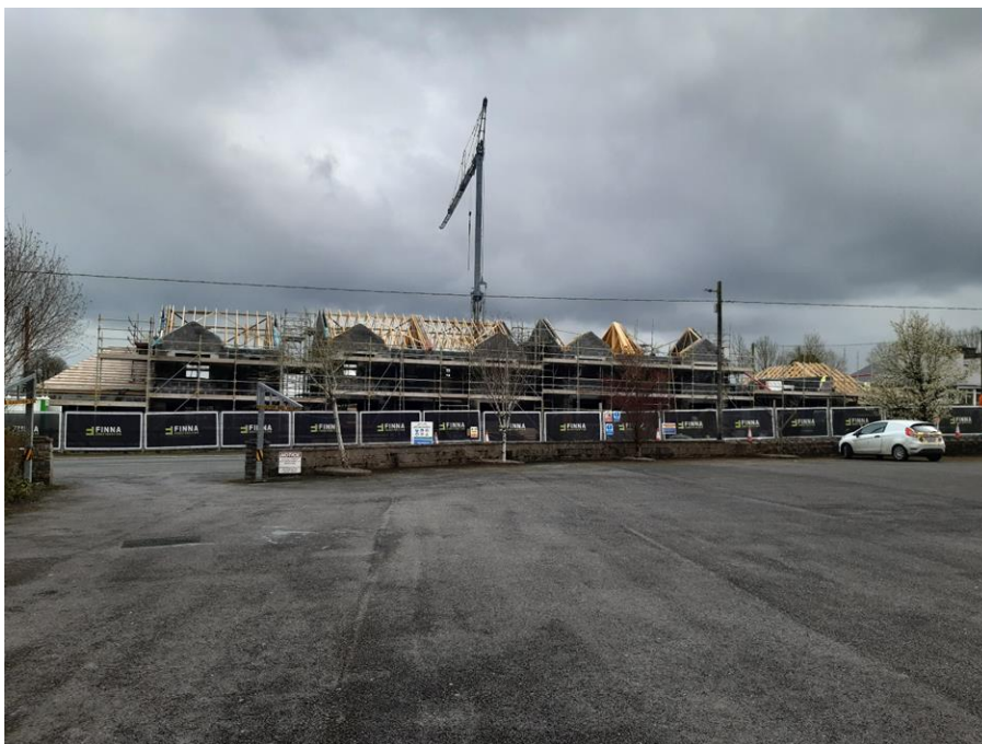
VIEW OF CONSTRUCTION WORKS AT PAIRC NA DARACH, AT BALLYMOE (APRIL 2024)
