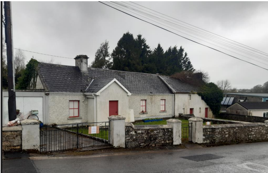
EXISTING DWELLINGS AND OUTBUILDINGS AT BARKHILL, WOODFORD
