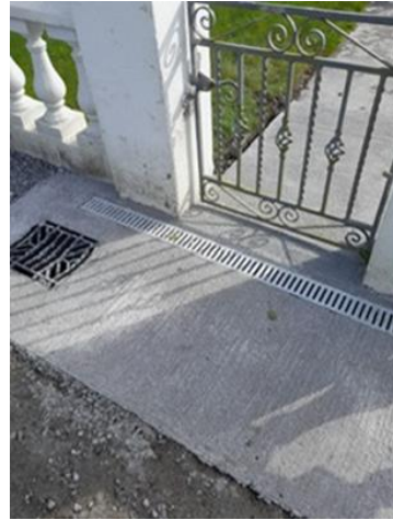
DRAINAGE WORKS AT KILCOOLEY ON THE N65 TO ALLEVIATE SURFACE WATER FLOODING
