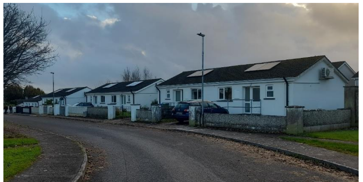
SINGLE STOREY DWELLINGS WITH EXTERNAL INSULATION, HEAT PUMPS AND SOLAR PANELS
