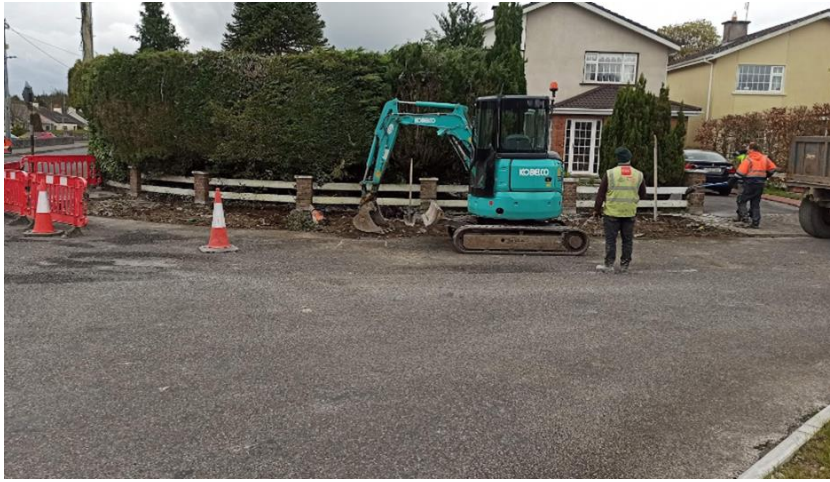
CAHEROYN DRIVE FOOTPATH UPGRADE
