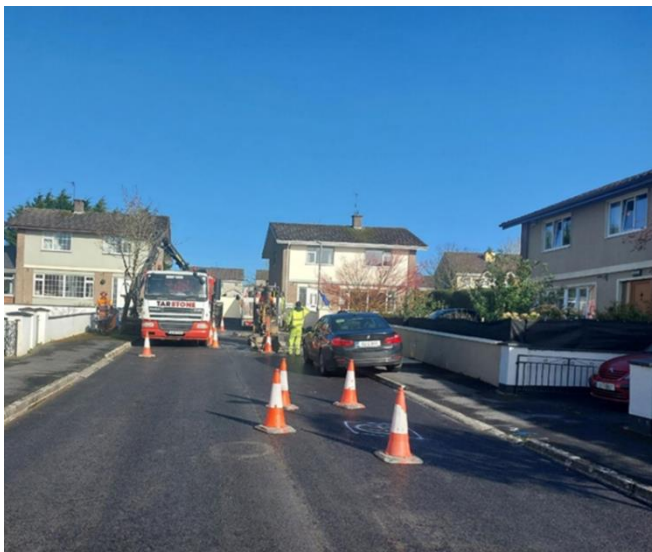
EXPOSING AND RESEATING IRONWORKS AT COSCORRIG CRESCENT FOLLOWING RECENT OVERLAY
