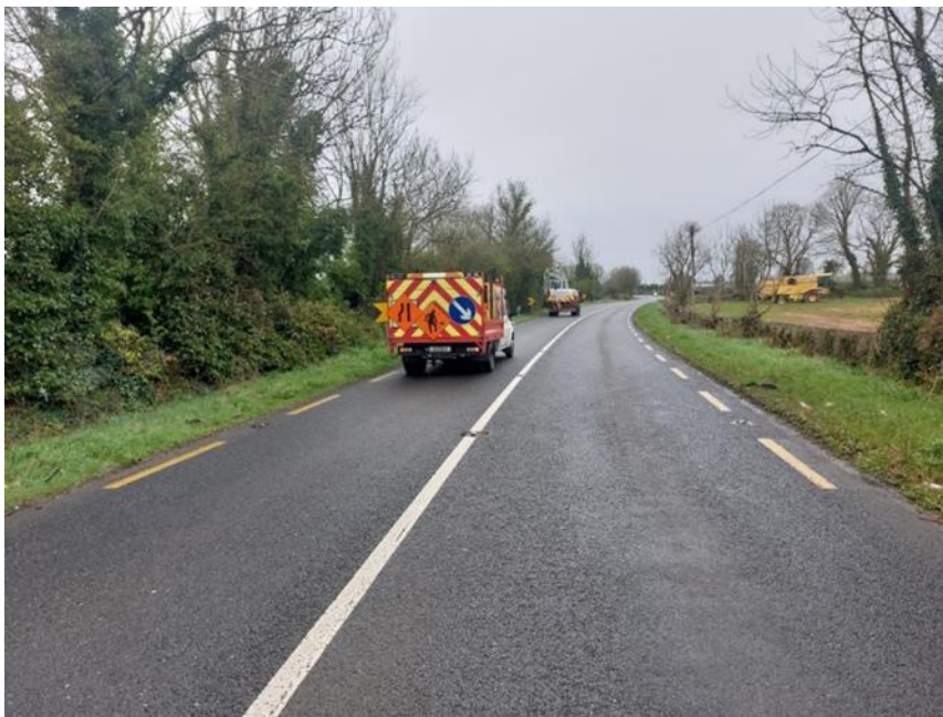
OPENING WATERTABLES ON THE REGIONAL ROADS
