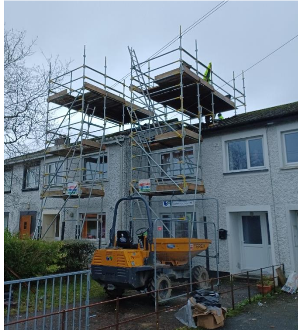
CHIMNEYS BEING DECOMMISSIONED & SOLAR PANELS BEING INSTALLED
